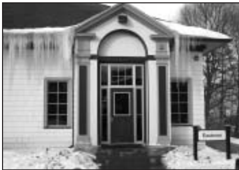
The outside of Eastman Hall is taking shape. A glass piece by local artist Nancy Gong will be installed soon.
