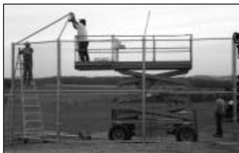
Workers put the finishing touches on the batter's cage.
